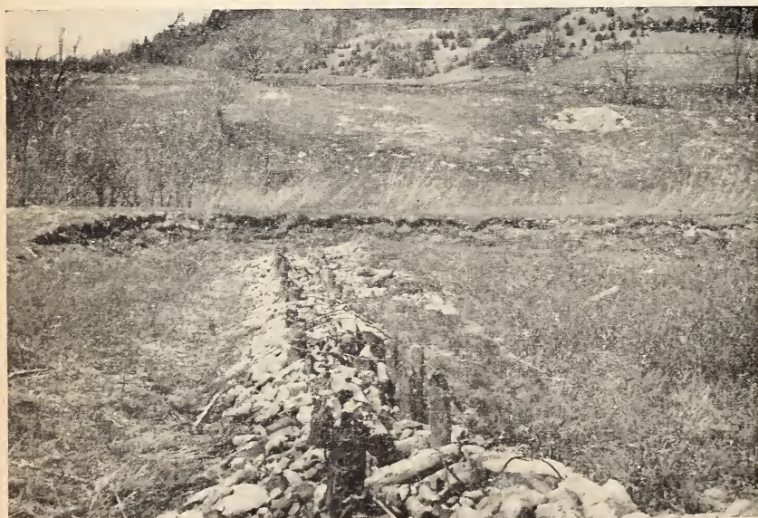
FIGURE 15.—New channel cut through plowed soil at farther end of check dam, 1946.
